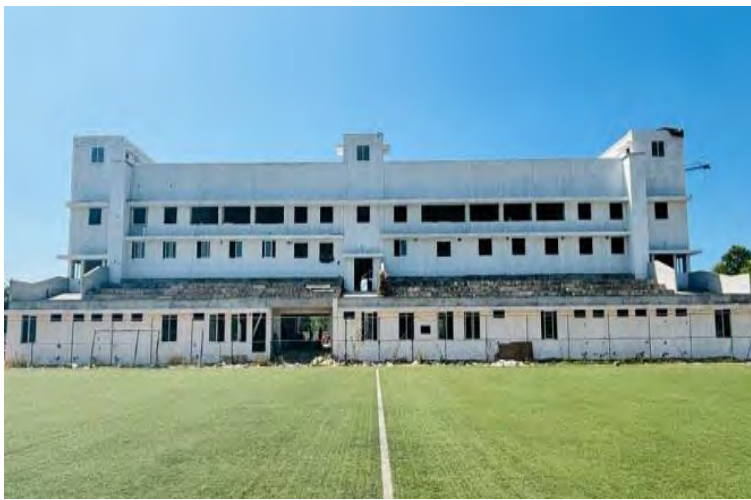
Fig 8.2 Pavilion gallery under construction
