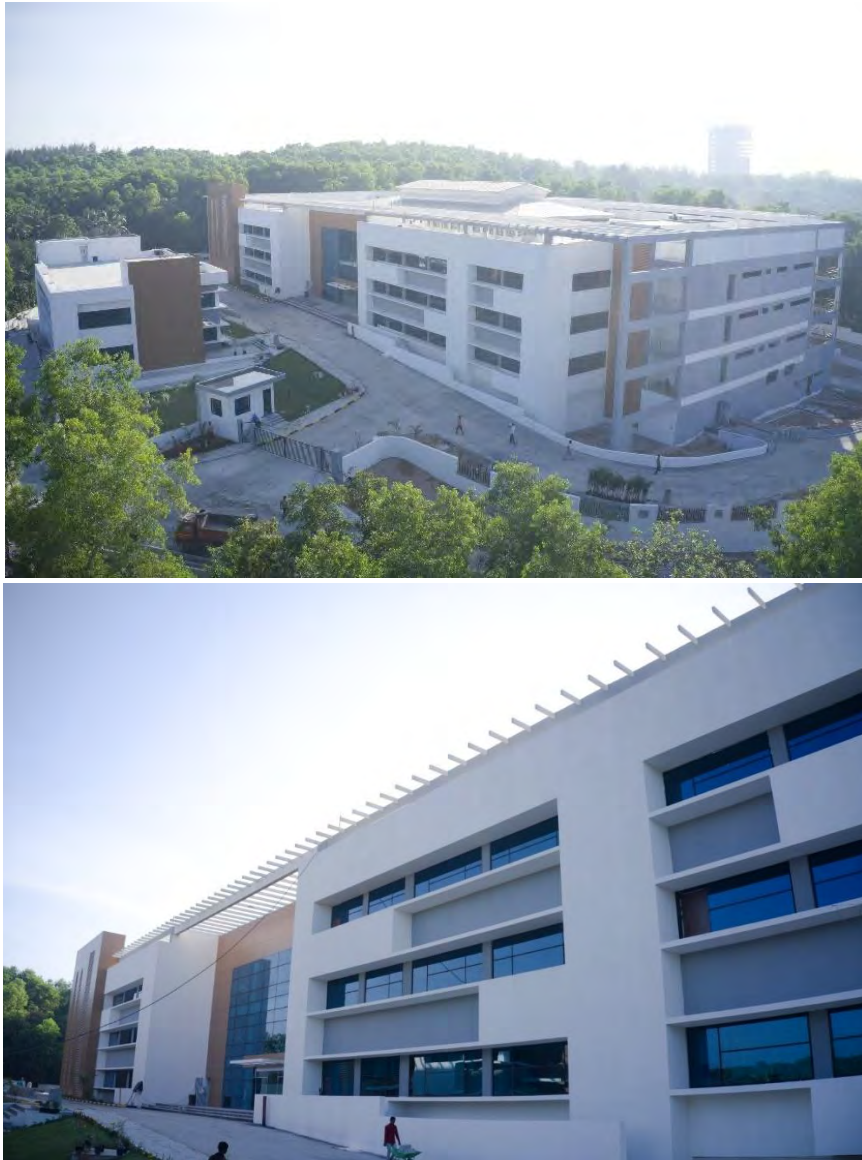
Fig 19.1 IT Building at Technocity
