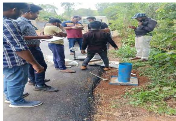
Field Dry Density (FDD) Test in shoulder
