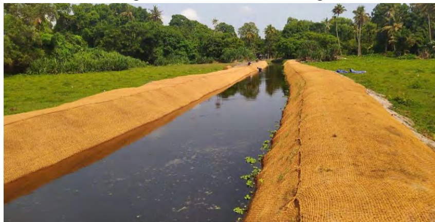
Fig 21.2 Phase II canal cleaning
