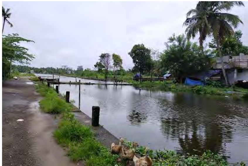
Fig 21.1 Phase I canal cleaning
