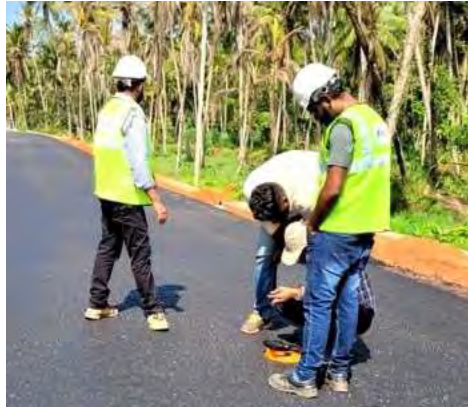
Asphalt Density Guage Tester at Perambra Bypass
