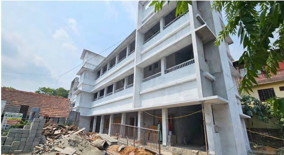
Fig 4.2 Academic block in progress
