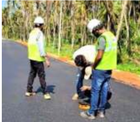
Asphalt Density Guage Tester at Perambra Bypass
