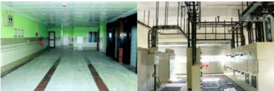
Fig 13.3 TH Payyanur – Interior view
