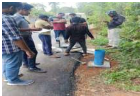
Field Dry Density (FDD) Test in shoulder
