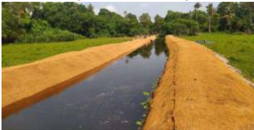
Fig 21.2 Phase II canal cleaning
