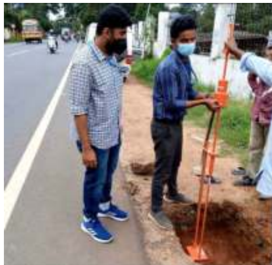
DCPT Test at Vazhimukku- Kaliyikkavila Road
