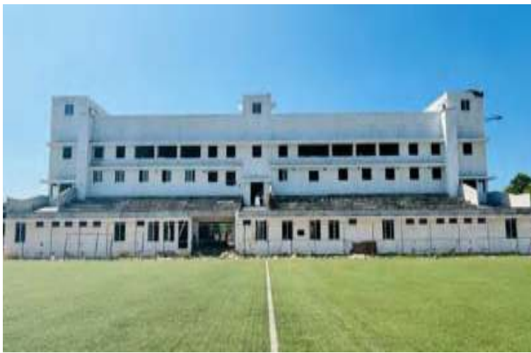
Fig 8.2 Pavilion gallery under construction
