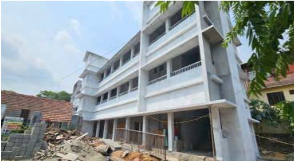
Fig 4.2 Academic block in progress
